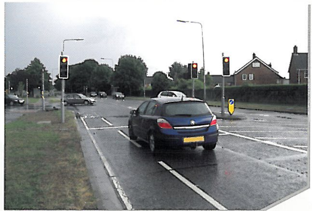
Western junction - after
